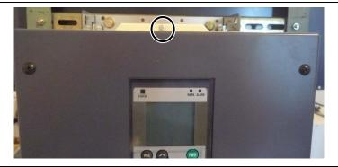
(2) Remove the two screws from the top of the fan casing.
